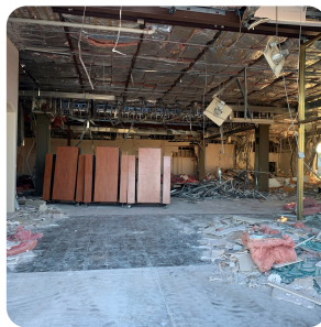
In November, renovations started on the Y's new branch, The Little Explorer's.
